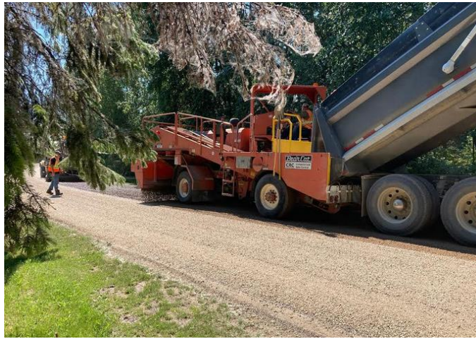
Chips being applied to oiled road
