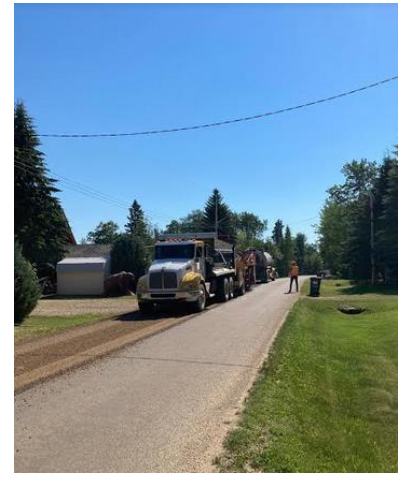
Chip sealing progress
